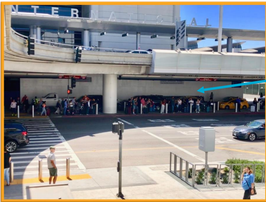
Terminal B, Arrivals Level New Construction Barricades
