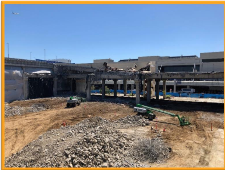
Parking Structure 3 / 4 Bridge Demolition
