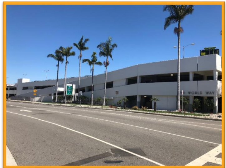
Parking Structure 7 Ramp Demolition
