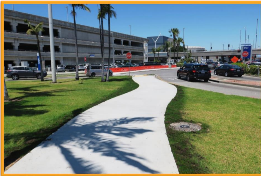
New Pedestrian Walkway Center Way, Facing Terminal 1
