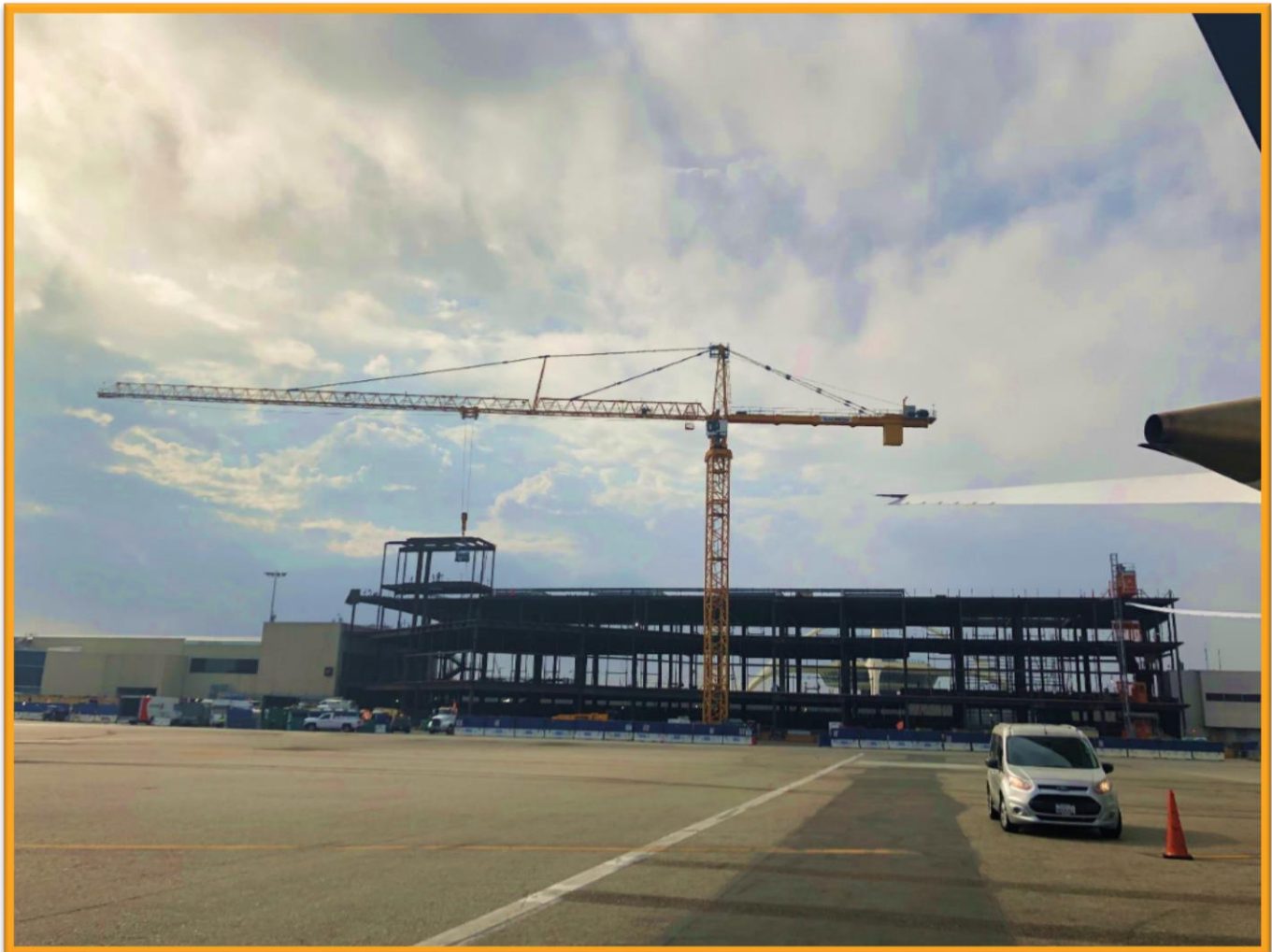
Terminal 1.5 Construction, Airside
