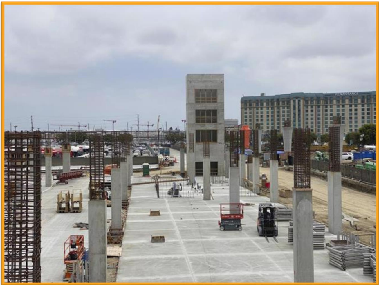
ITF-West Construction Site located between Westchester Parkway and 96th Street
