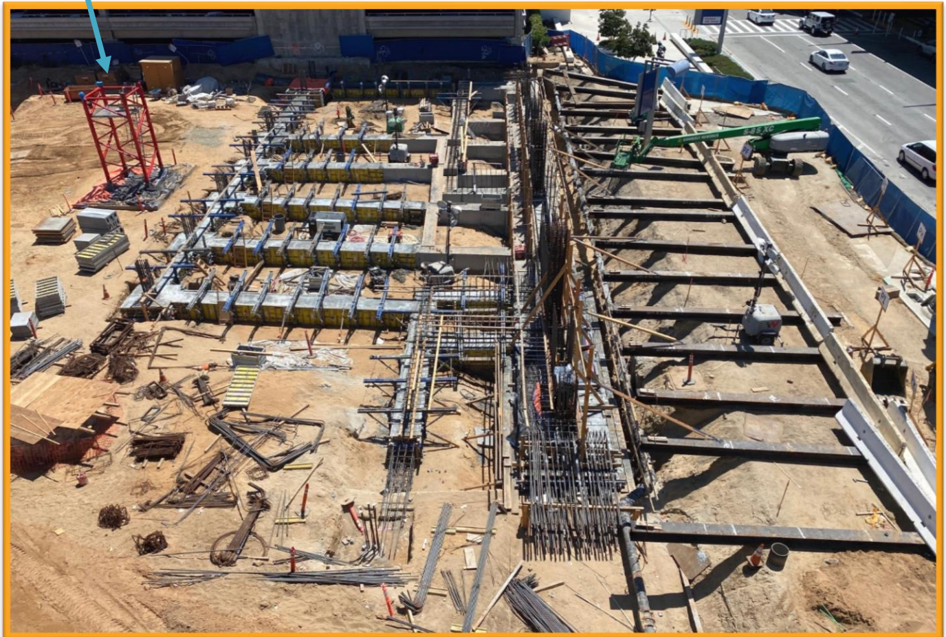
APM West Station construction between Parking Structures 3 & 4
